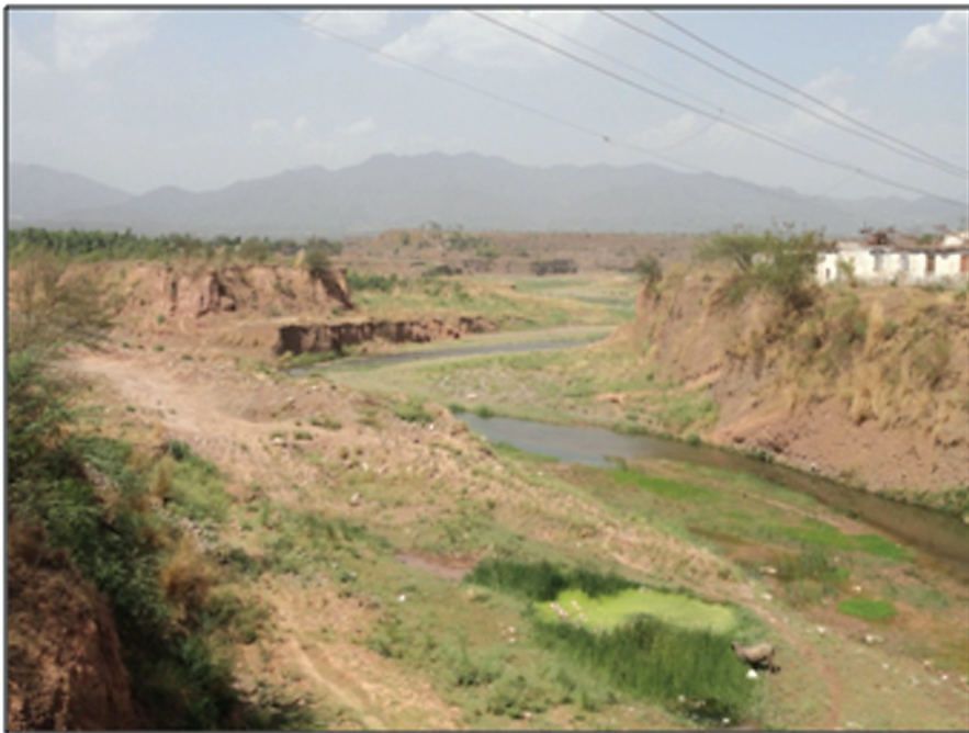
Plate B: Stream bank erosion by Kaushalya River (see page 59)
